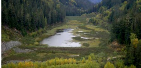
Example of reclaimed tailings impoundment developing as a wetland, Snip Lake, BC
