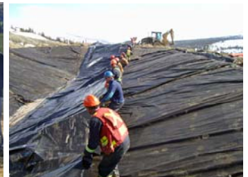
L to R: drumming ceremony, crews installing sump liner
