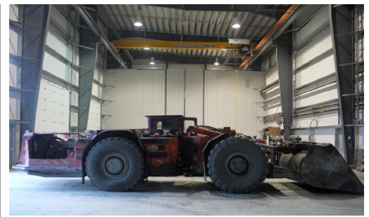
Truck shop with radiant heat floor
